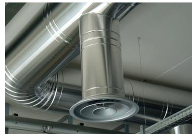
**Fig. 2** Special air diffuser for cast shop conditioning system
